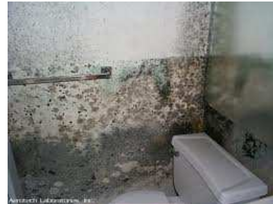
Cladosporium, Aspergillus, and Penicillium on painted dry wall surface (acmeflood.com)
